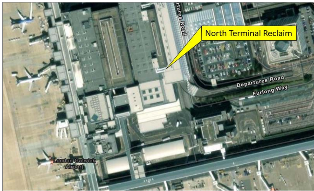
Figure 43: Location of North Terminal Reclaim
